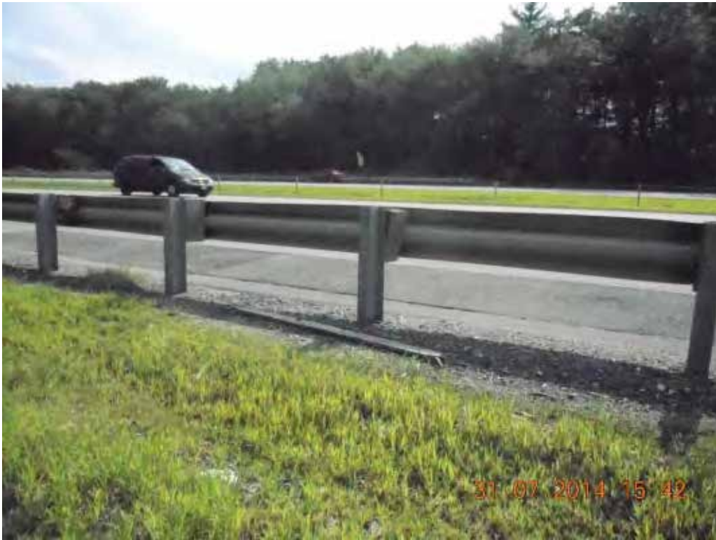
Route 3 Looking West Towards Old Concord Road
