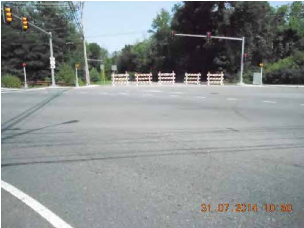
Middlesex Tpke and Concord Road Intersection
