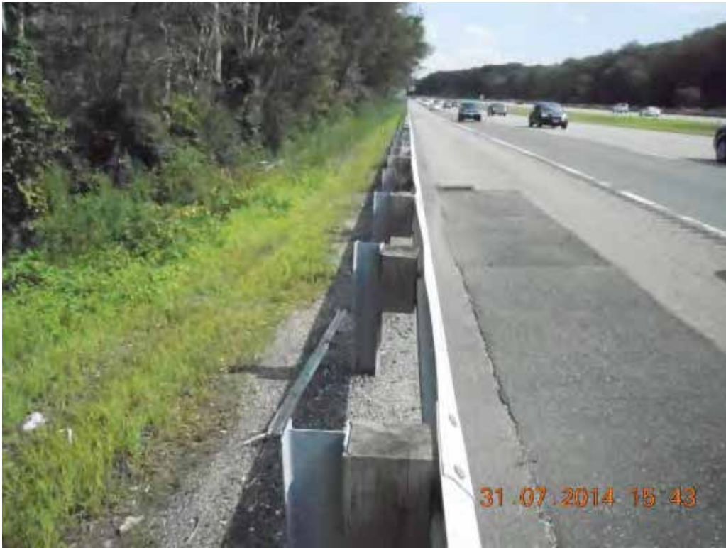
Route 3 Looking South
