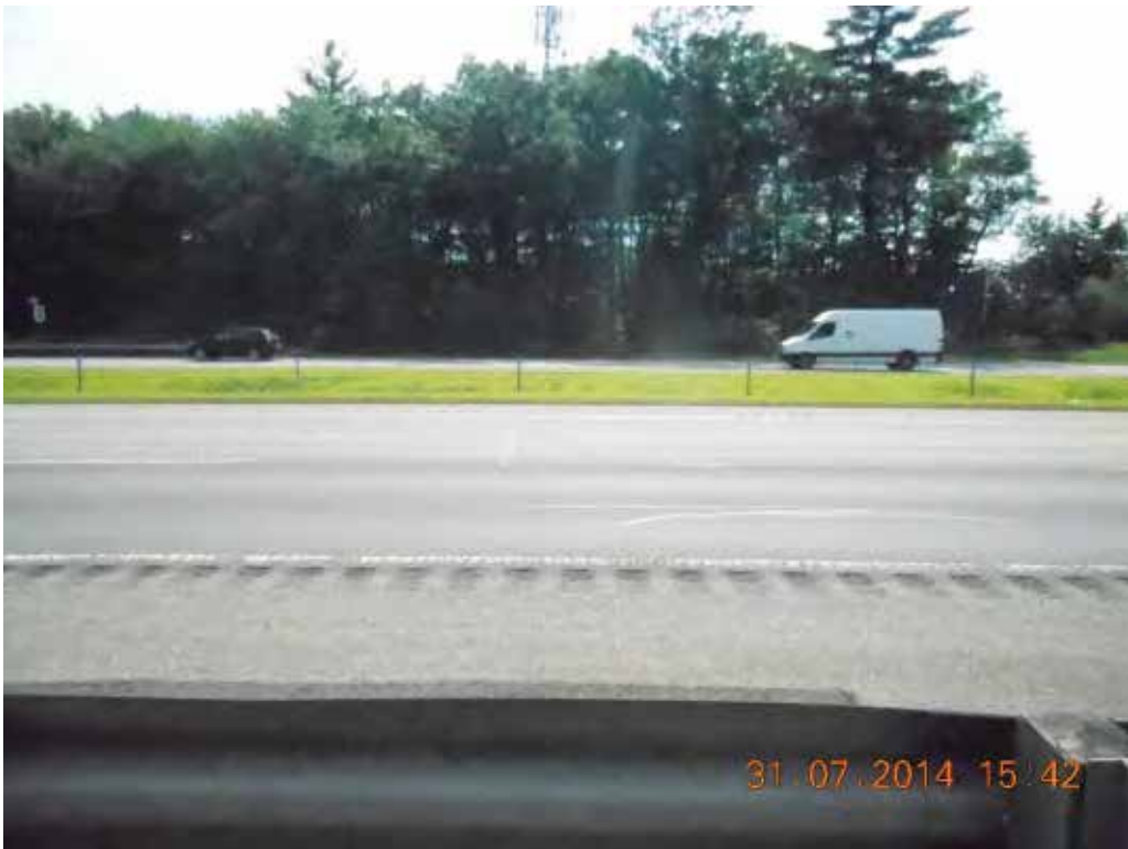
Route 3 Looking West Towards Old Concord Road
