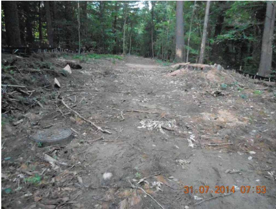
18'± Wide Gravel/Dirt Road Segment Parallel to the Concord River
