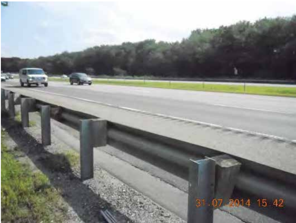
Route 3 Looking West Towards Old Concord Road
