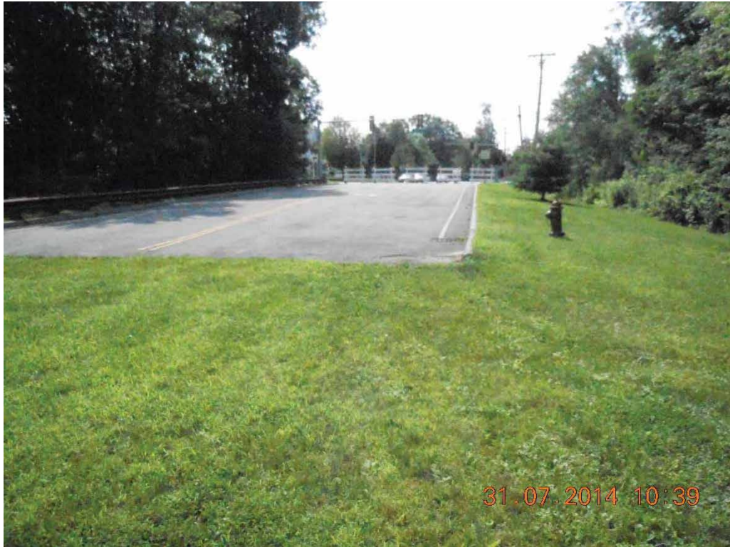
Dead End Segment of Middlesex Turnpike
