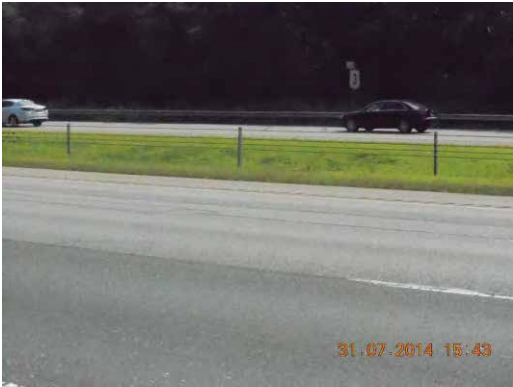
Route 3 Looking West Towards Old Concord Road
