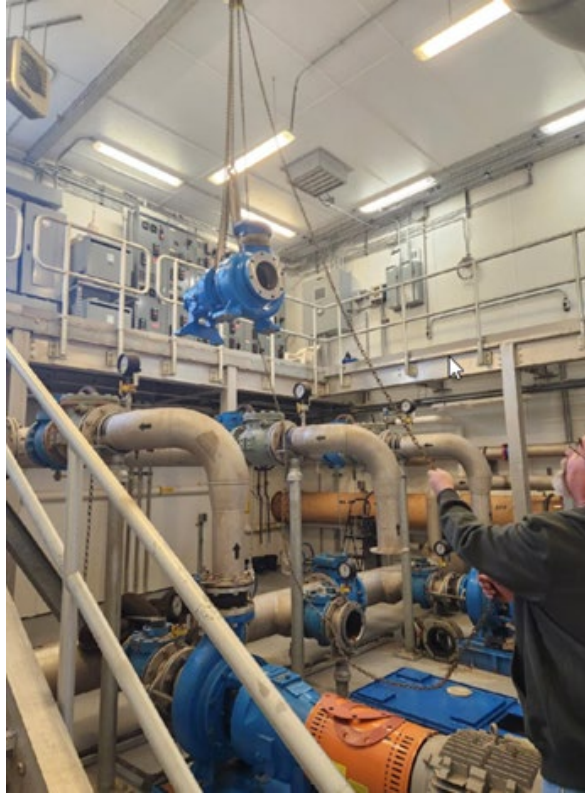
Comag RAS Pump being lowered into place
