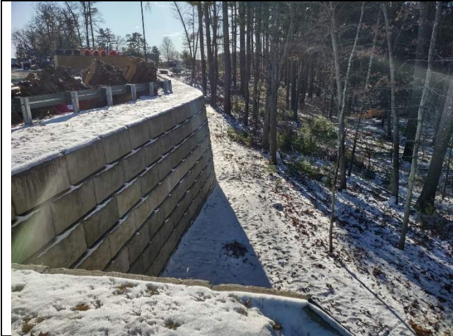
Photo 5: Existing Concrete Block Wall
