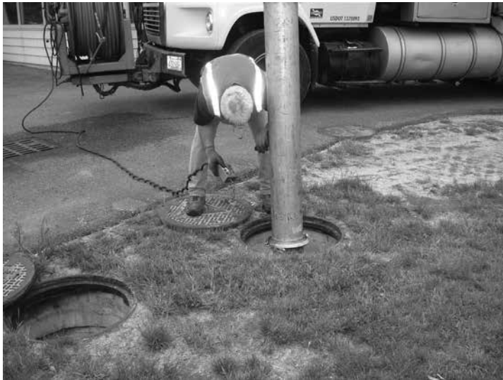
A Cascade Separator unit can be easily cleaned in less than 30 minutes.
