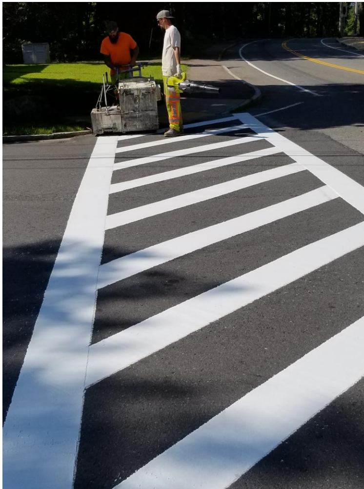
The Highway Division installed over 200 thermoplastic crosswalks last spring/summer.
