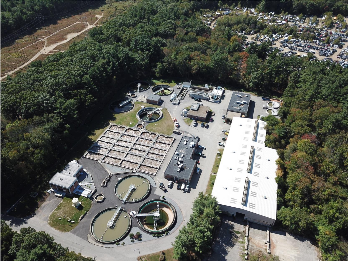
Drone flyover of the Wastewater Plant
