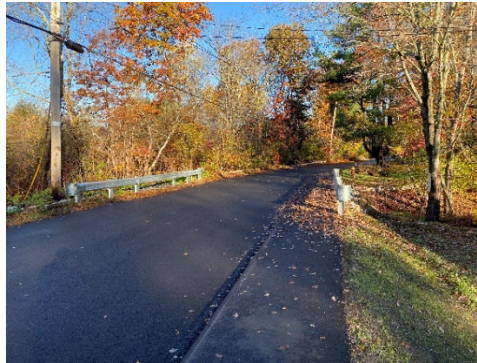
French Street paving and new sidewalk
