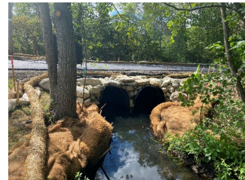
French Street culvert-completed by DPW
