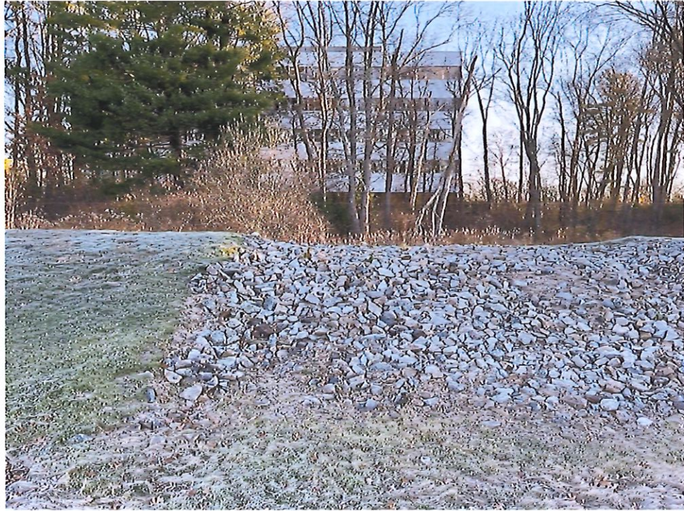
Image 3: Existing Basin Rip Rap Spillway
