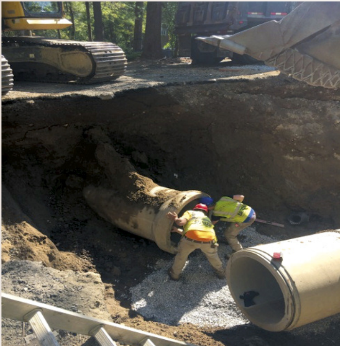
Sumac Street culvert installation.
