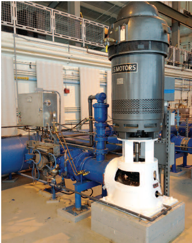
5 million gallon per day finished water pump.
