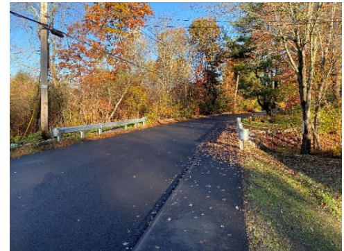
French Street paving and new sidewalk
