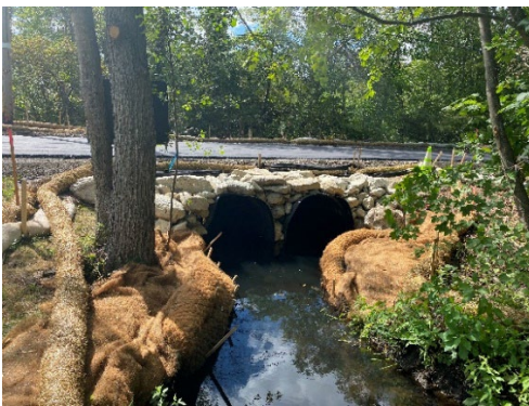
French Street culvert-completed by DPW
