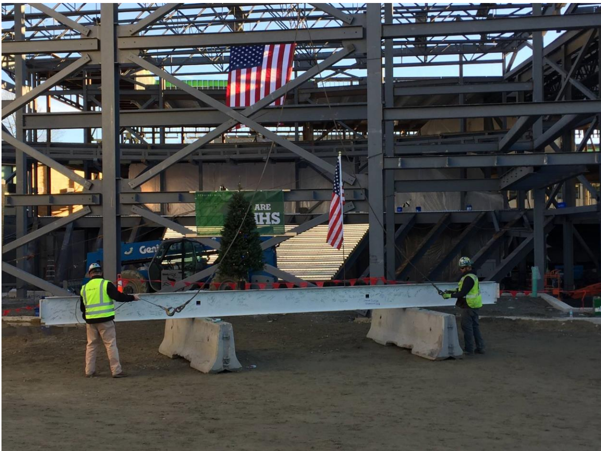
The final beam for the new Billerica Memorial High School
